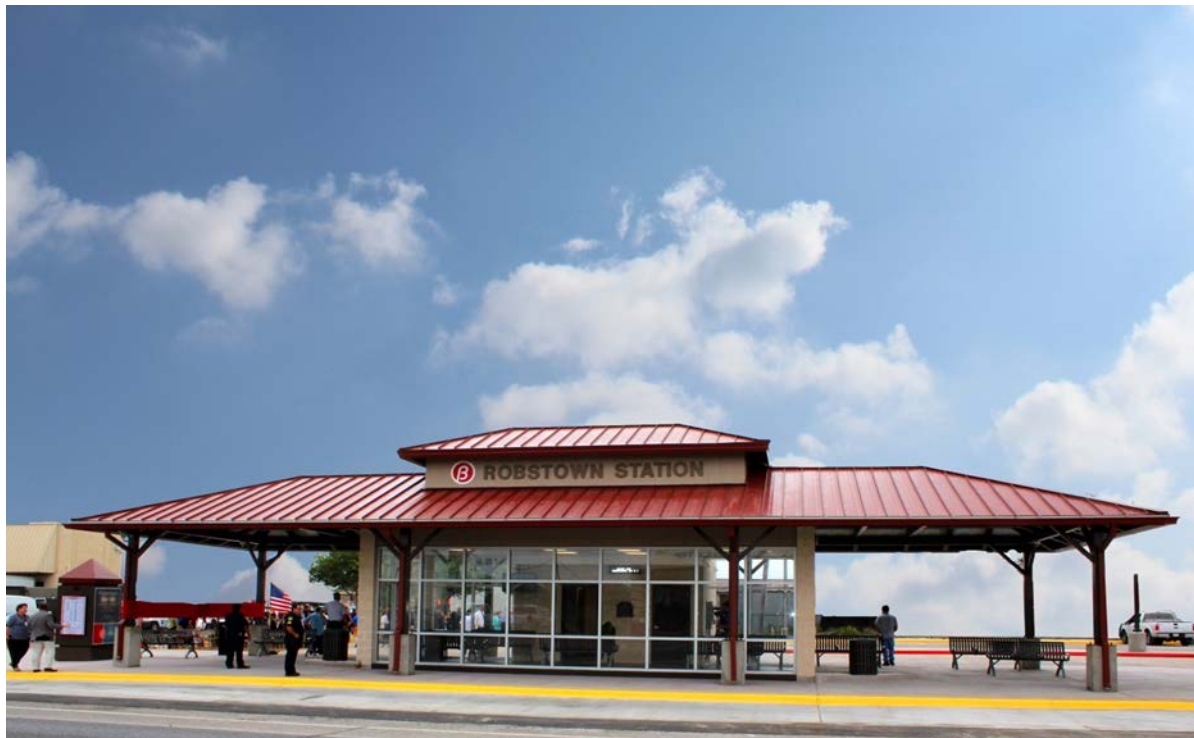
Robstown Transfer Station
