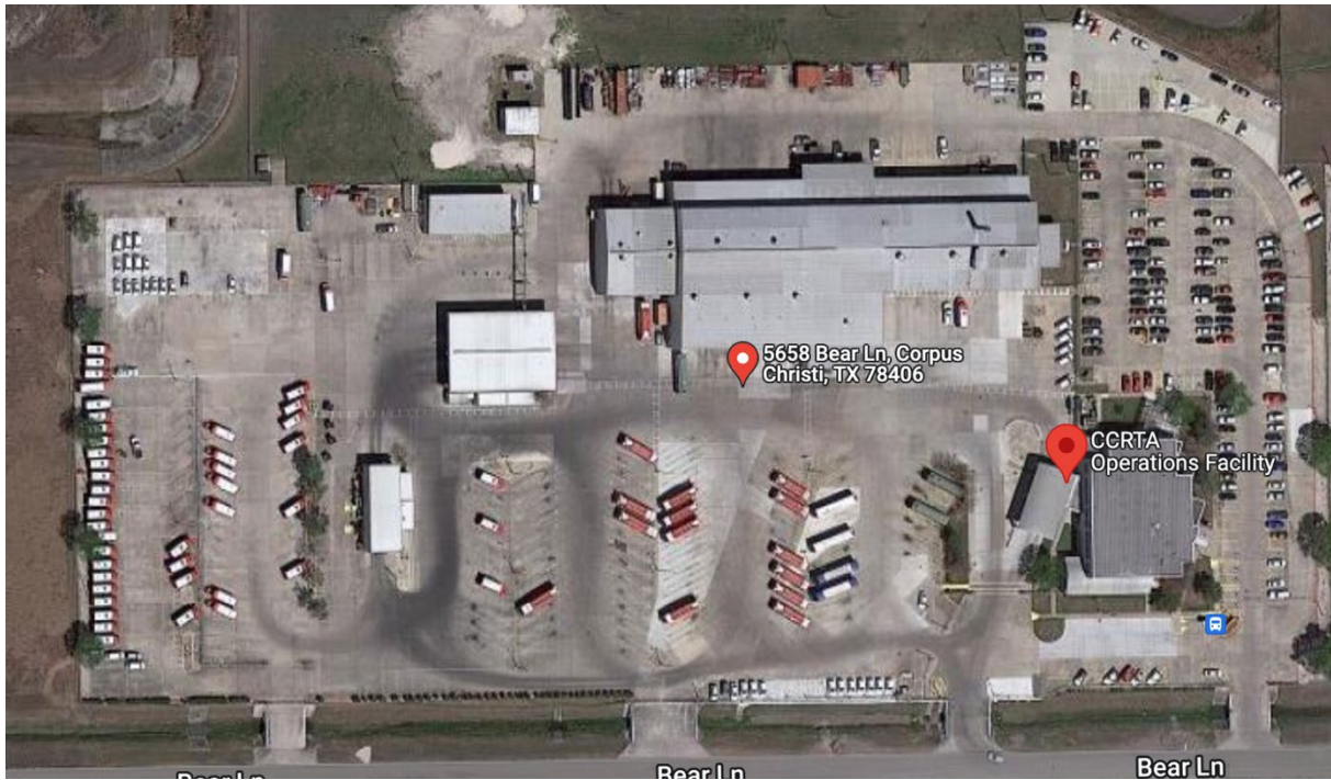
Figure 4 - CCRTA Operations and Maintenance Facility
